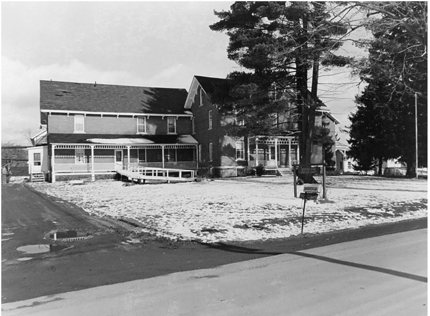
Main Building, Cortland County Poor Farm, Cortland, New York. Robert Gailor, Jr., December, 1981. Looking northeast from Loring Crossing Road at west wing and central unit. Courtesy of the Cortland County Historical Society.
