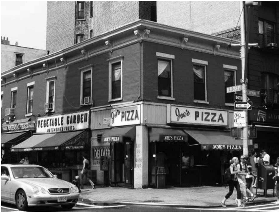
Corner building at Bleecker and Carmine, home to Vegetable Garden and Joe's Pizza. Photo courtesy of Jennifer De Ornelas Nobriga.
