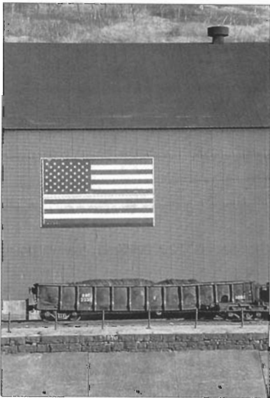
Bar, Rod, and Wire Division, Bethlehem Steel Lower Works, Johnstown, PA. Photo by James W. Harris
